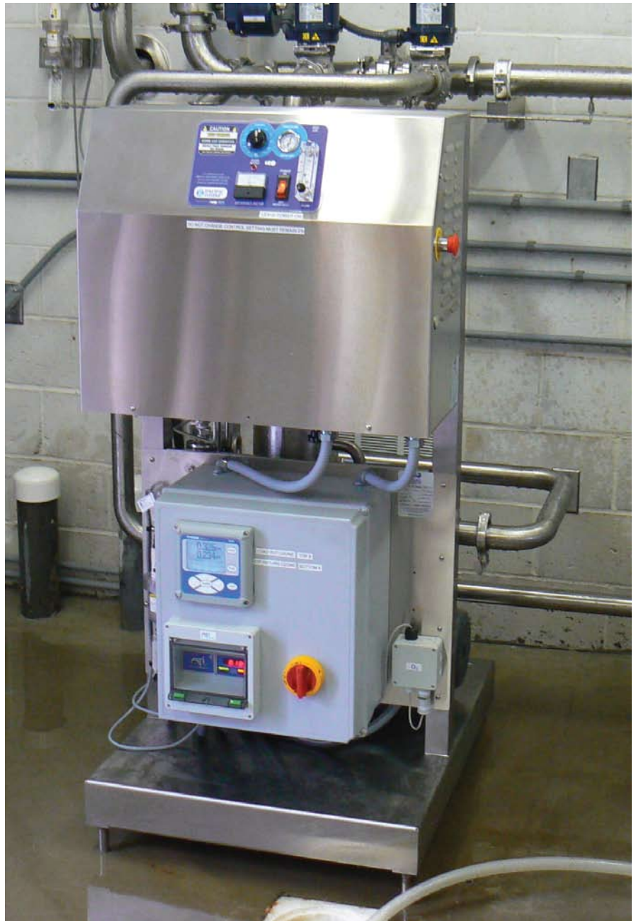
An SGC22 Ozone Generator System powers a Horizon 060 Integrated Ozone System at a remote spring water collection site.
