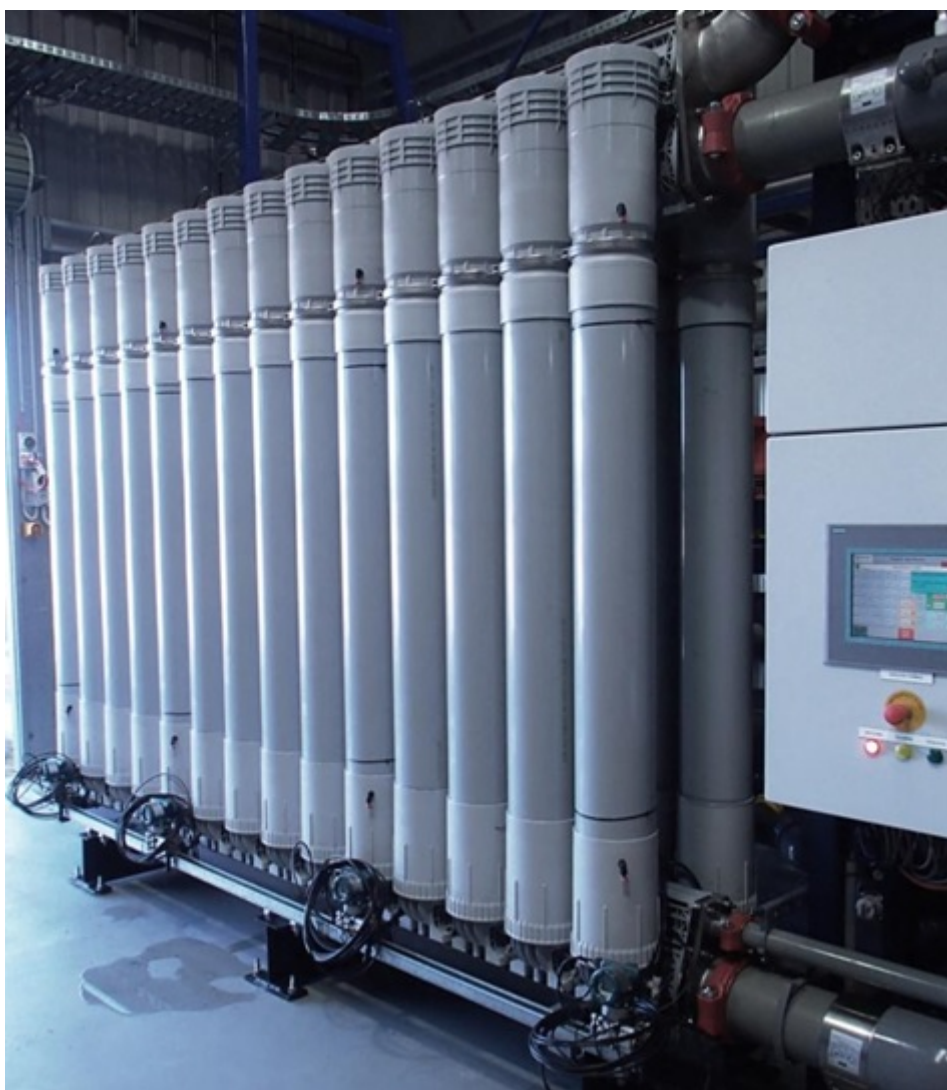
Typical MEMCOR® CPII MemRACK installation
