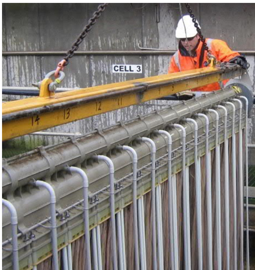
Figure 1: Typical MemRACK™ MBR nylon Rack Assembly suspended from a Rack Lifting Beam (yellow).
